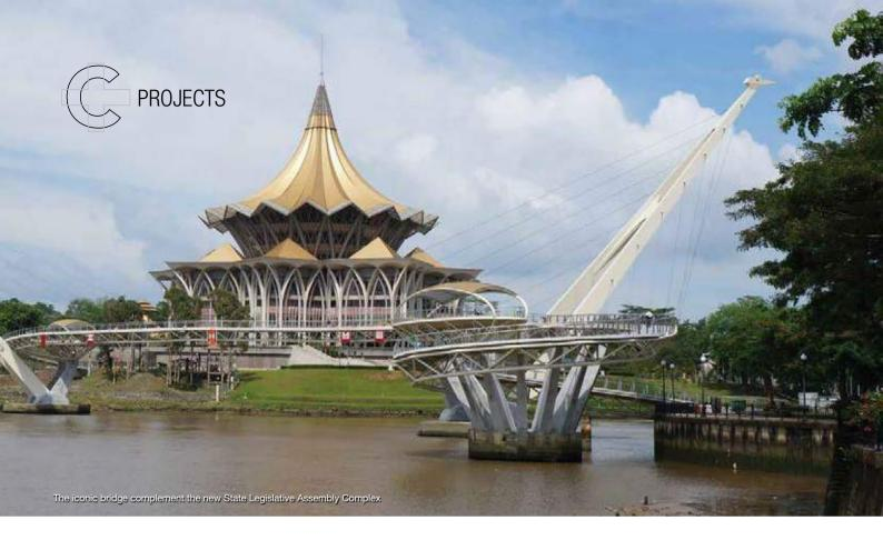
3.25-metre-wide walkway that meanders 335 metres over the Sarawak River. Its curved plan allows a comfortable walkway gradient that is suitable for access by disabled persons, while still providing sufficient clearance for river vessels to pass beneath it. It also orients the bridge towards particularly attractive surrounding viewpoints.
