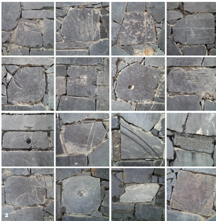
1 Axonometric diagram of the project's programme 2 Wall segments made from debris and discarded stones from Kem Trong 3 Conceptual drawing
