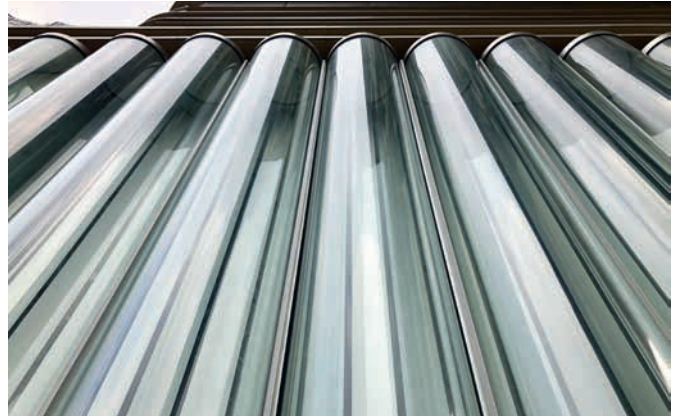
The 9m high glass tube façade for K11 Museum with integrated CCF system was the first built in Asia. © seele
