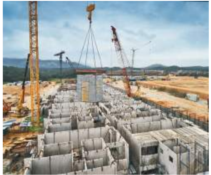
Just ‘plug and play’: No wet works required with the bathroom pods
