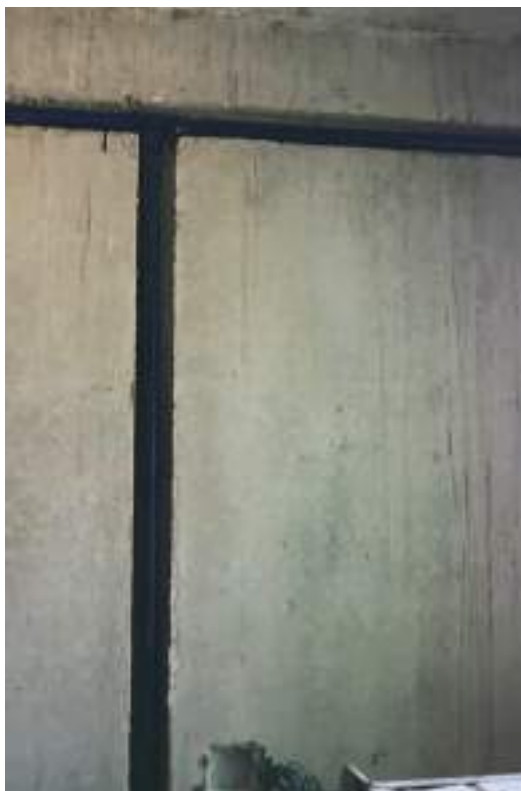
No more hacking with cast-in grooves for pipes
