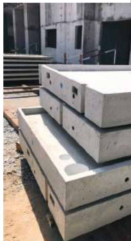
Seamless bathroom trays prevent leakages
