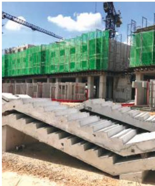
Prefabricated staircases waiting to be installed
