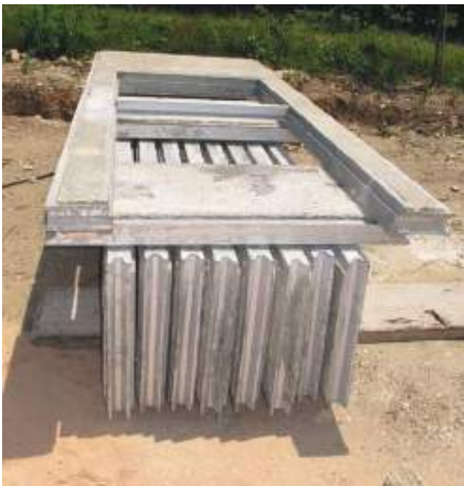
Large-size Kenafibre panels ready for installation
