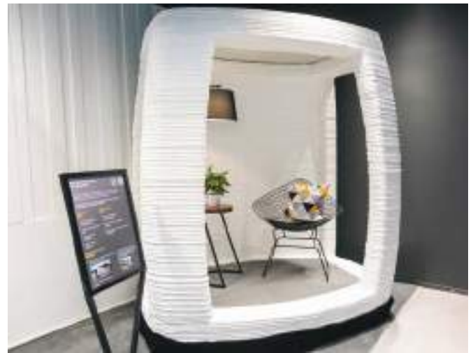
3D-Printed Concrete Structure
