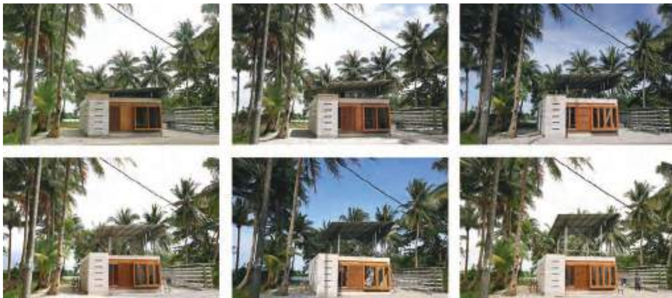
Hoisting the roof of the Rumah Tambah, or expandable house, in Batam: a sustainable housing unit
