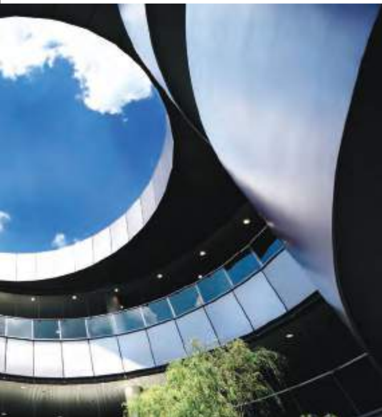
Aluminium sunscreens reduce solar glare and keep rain out
