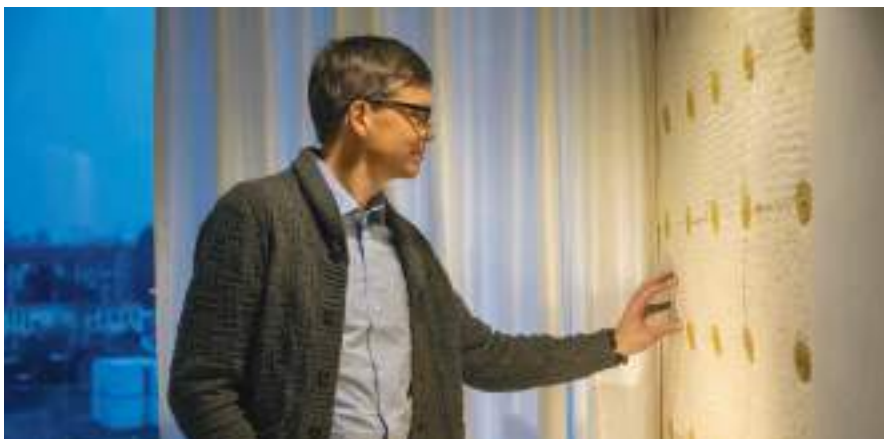
The UMAR unit by Werner Sobek with Dirk E. Hebel and Felix Heisel applied and tested mycelium-bound building elements as wall insulation
