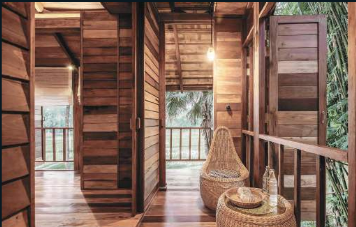
Double-layered façade acts as an insulator against extreme heat
