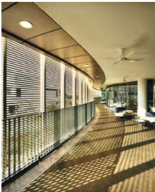
Aluminium sunscreens reduce solar glare and keep rain out
