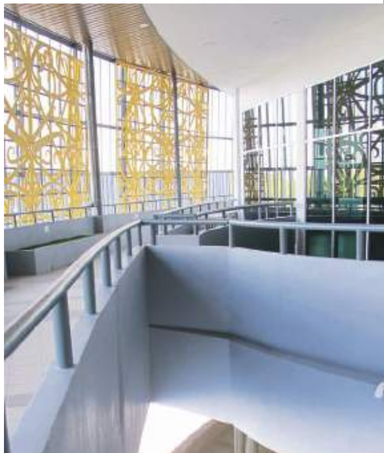
Slab cut-outs allow cool air from the pond below to circulate in building
